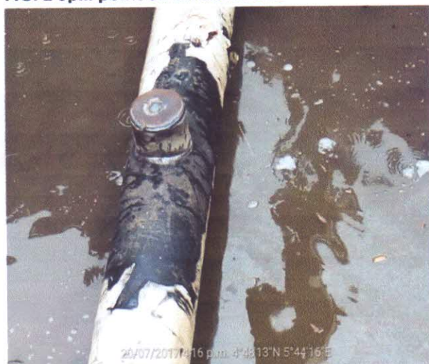
FIG 3: Coning of spill point
